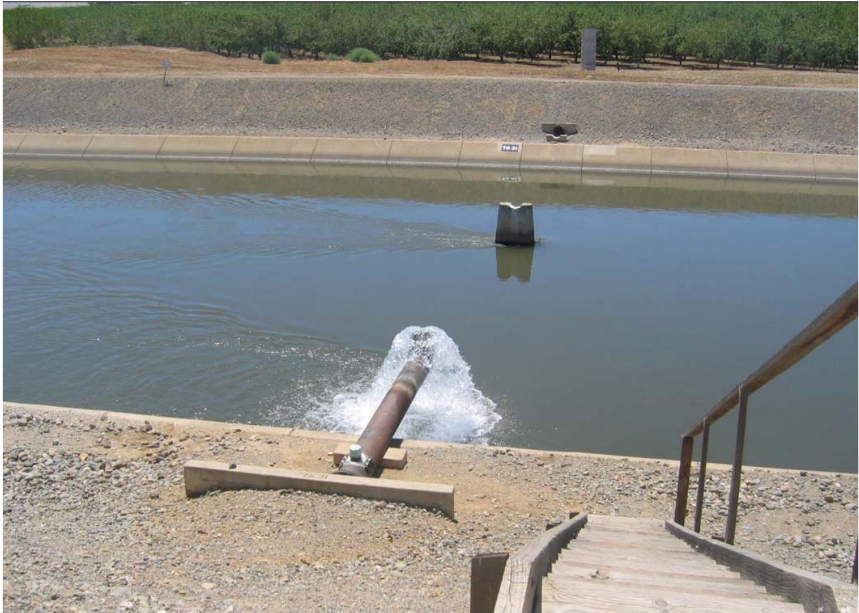
Groundwater Pumped into the DMC near Los Banos, California U.S. Department of the Interior Bureau of Reclamation Mid-Pacific Region August 21, 2008
